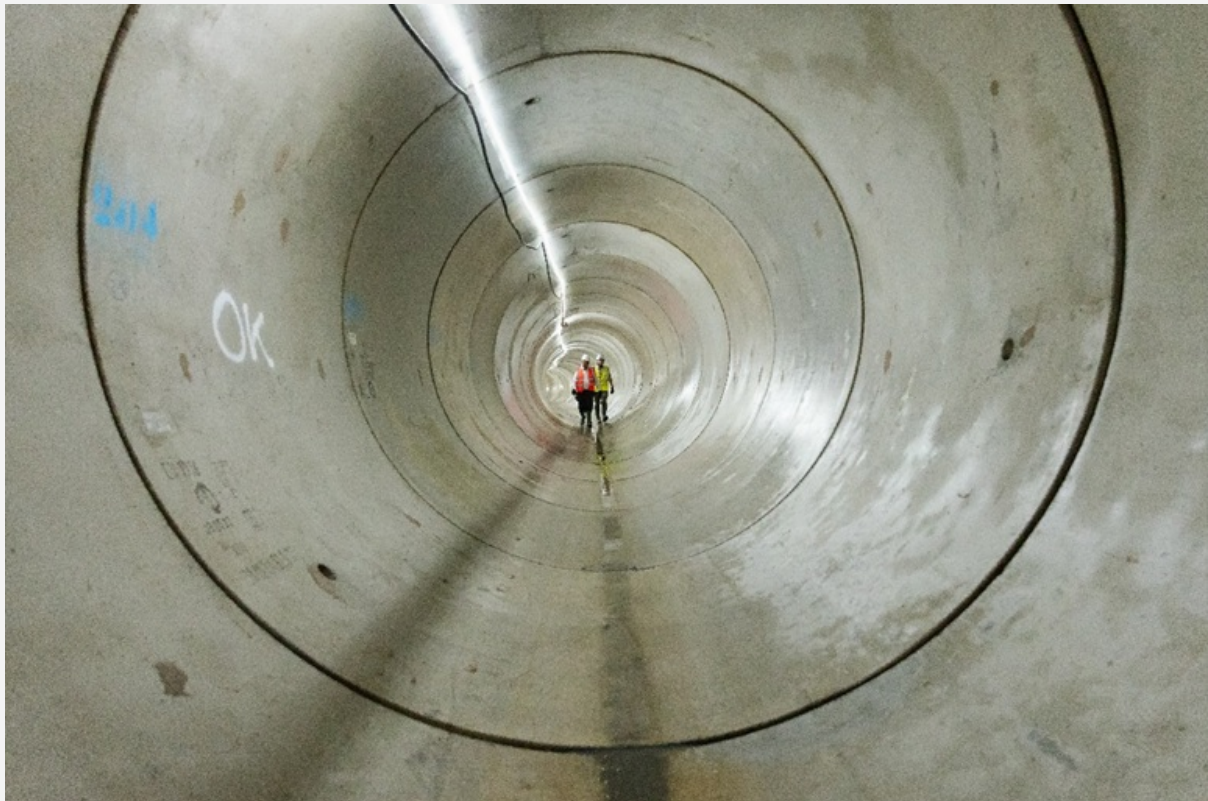
Figure 6. Austerlitz rainwater storage basin — intercepting tunnel
